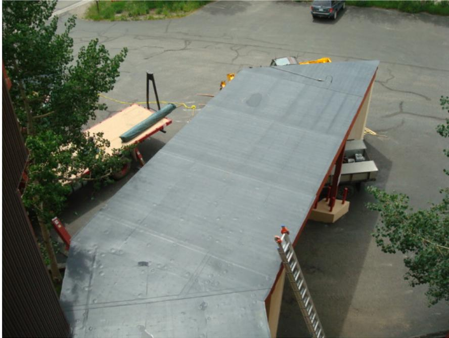
Photo 4: Bird's eye view of the finished product on the porte-cochere. Small air bubbles can be seen on the left side of the roof, but these occur regularly when installing a roof like this and disappear after several days.
