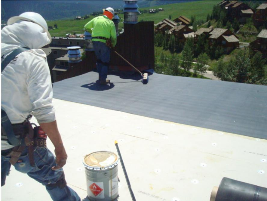
Photo 8: The EPDM layer that was shown getting glued on in the above pictures when finished.
