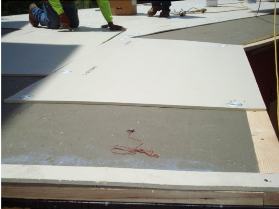
Photo 2: Here the installation of the sub-roof materials over the porte-cochere is shown. This roof was completely replaced after their first day of work. In this picture as well as several below, the circular silver disks that are being used to mechanically fasten the insulation and cover board can be seen. The hold down the roof and then the EPDM layer is glue on top of that.
