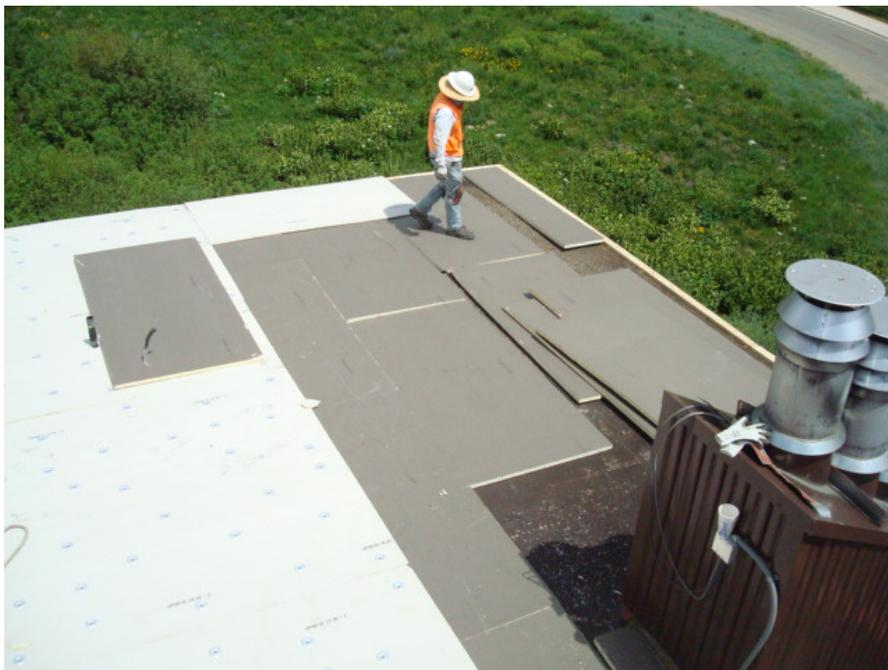
Photo 5: This is the installation of sub-roof materials on the south side of the building. Here you can see the bottom gray layer of insulation as well as the top white layer of insulation.
