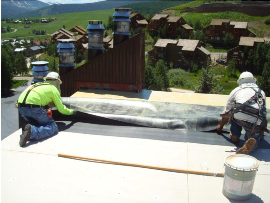
Photo 6: The Carlisle roofing membrane is glued on top of the insulation layers on the southwest corner of the building. Glue is placed on the insulation layer as well as the EPDM roof membrane layer.
