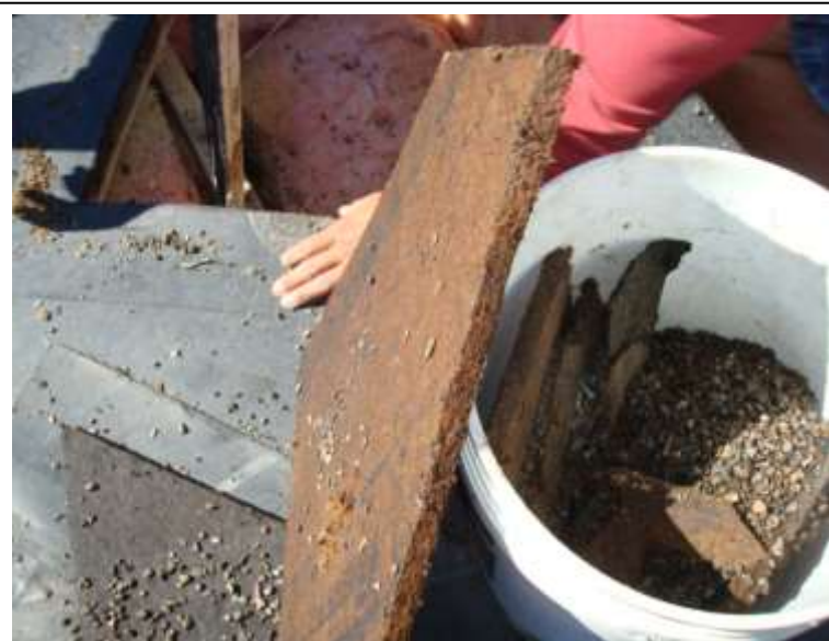
Same location as photo 23. Can't really tell in this photo but the underlayment board is completely saturated with water. Underside of Plywood, roof joist and insulation are dry.
