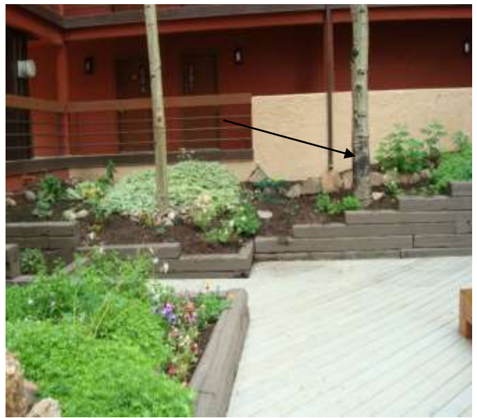
Roof downspout could bring significant water to this area. Is this problematic? Other downspouts could potentially drain water to areas where not wanted. This will be studied further as part of the building and grounds assessment.
