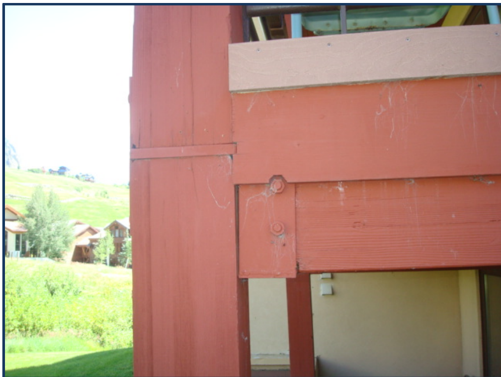
Photo 8: Existing Splice in Column #5
